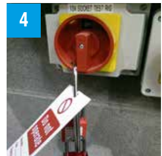
4. Application of Lockout/tagout devices
